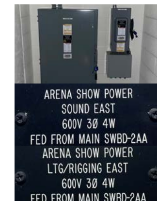
3rd Floor East
