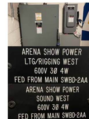
3rd Floor NW Corner
