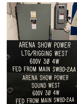
3rd Floor NW Corner
